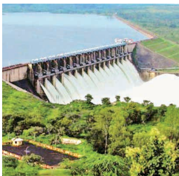
Mahi Dam is one of the key sources of potable water in the area.
