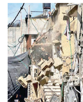
Damage following an Israeli raid on Sunday.
