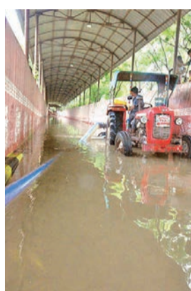
Water pumps being used to drain the JK colony underpass which was almost submerged.
