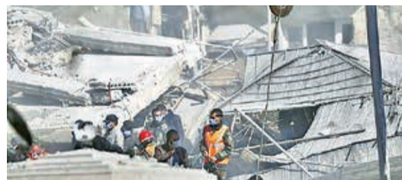
Emergency services work at a building hit by an air strike in Damascus, Syria, on Saturday. PTI
