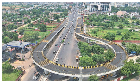
The clover leaf at B2 bypass will help in facilitating smooth traffic movement and will provide relief to general public.
