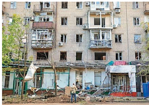
The mangled remains of the building after the attack.
