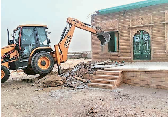
A religious structure is being demolished by the authorities under Operation ‘Border Clean’ in Jaisalmer, on Thursday.
