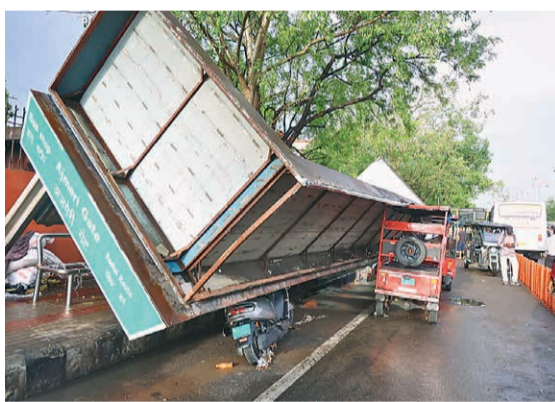
Ajmeri Gate Bus Stop shelter collapses during rain, trapping several vehicles underneath in Jaipur, on Thursday.
