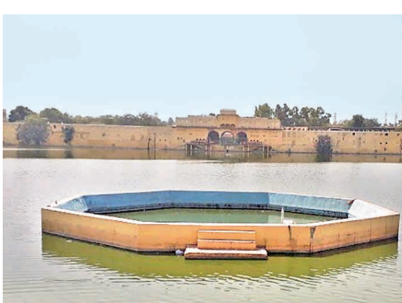
Rajasthan Tourism Development Corporation had handed over the project to the Smart City Project but no action was taken to get the maintenance done by the contract firm. FILE
