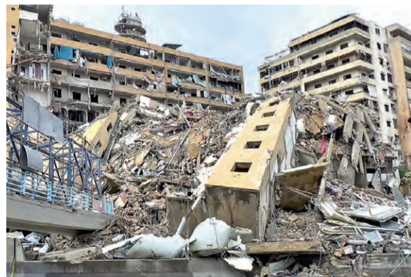
A destroyed building that was hit in an Israeli airstrike in Dahiyeh, in the southern suburb of Beirut, Lebanon. PTI
