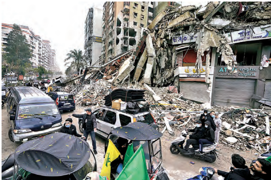
Displaced residents return to Dahiyeh, in Beirut, Lebanon, following a ceasefire between Israel and Hezbollah that went into effect on Wednesday.
