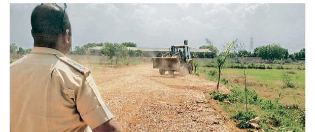
JDA bulldozer razing illegal construction in Jaipur on Monday.
