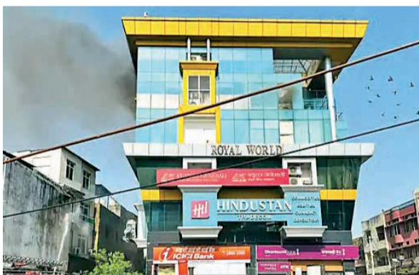
The building was evacuated by first responders as fire spread across fourth & fifth floors on Wednesday. SANTOSH SHARMA
