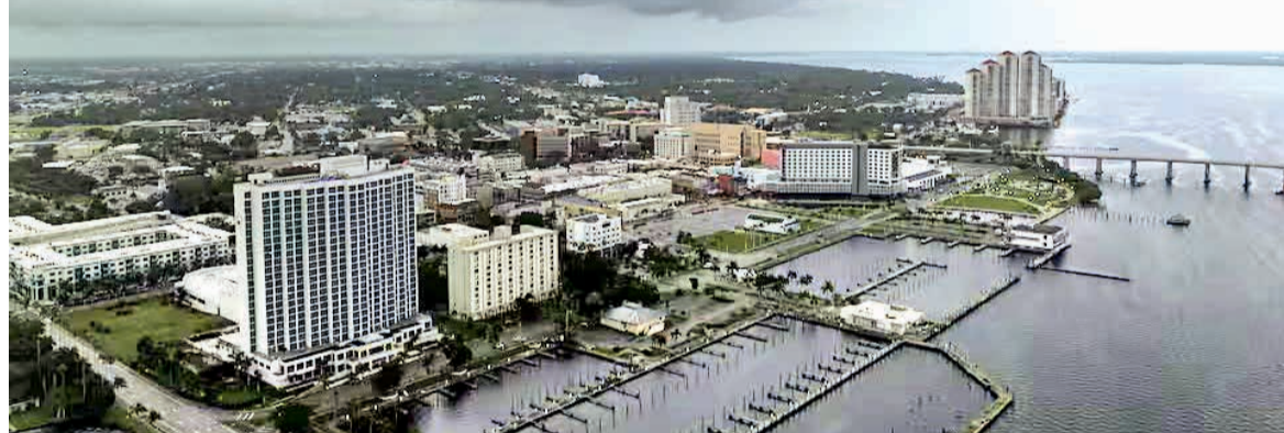
A drone view shows storm clouds over the Caloosahatchee River as Hurricane Milton approaches Fort Myers, Florida, U.S. President Joe Biden warns of "worst" natural disaster in a century. Hurricane Milton To Bring Water Surge Of Up To 15 Feet To Tampa Bay.
