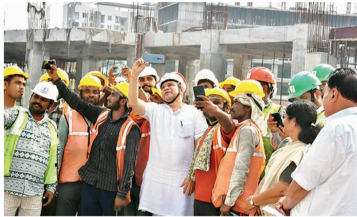
Ashwini Vaishnaw takes selfie with workers during an inspection visit of the under-construction Gandhinagar Railway Station in Jaipur on Tuesday. NAIM KHAN
